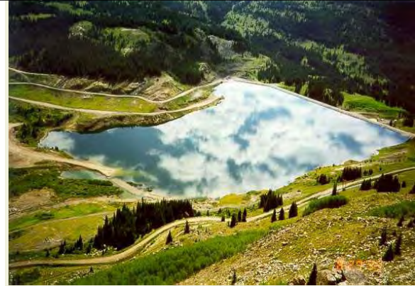
The Eagle Park Reservoir, which formerly contained tailings and impacted process water, was reclaimed in the 1990s.
