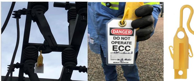
Power Line Jumpers – A removed jumper, and when a power line has been properly tested and grounded is an acceptable means of de-energizing the powerline for work to take place. This air gaps the line being worked on from the energized system.
