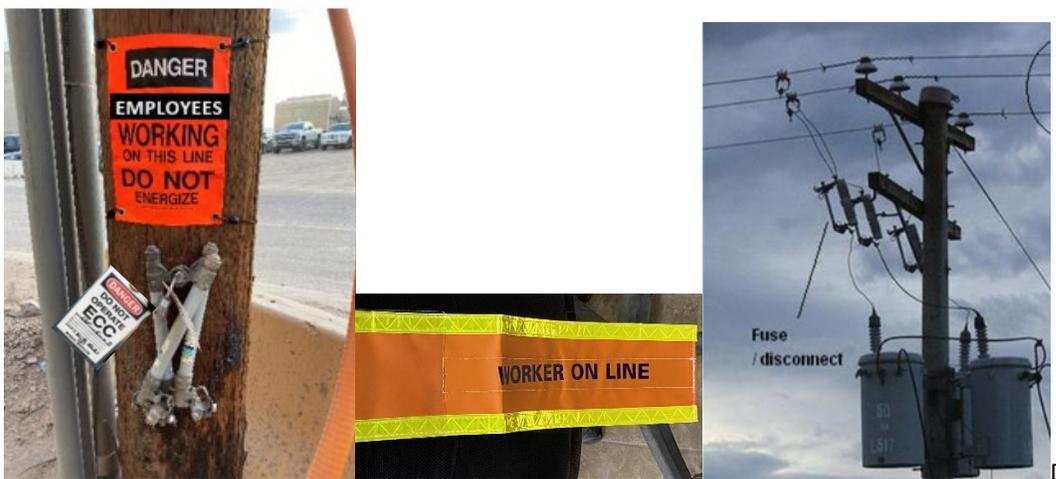
Blade Cut Outs- The use of blade cut outs is an acceptable method for isolating electrical energy from equipment when the following actions are met:
