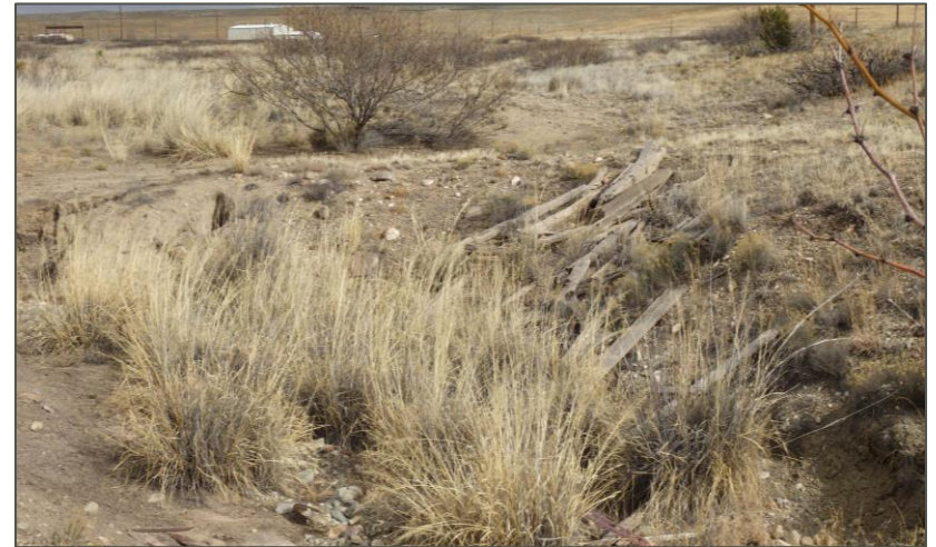
January 2020. East headcut at Edwards Ranch. Looking upstream.
