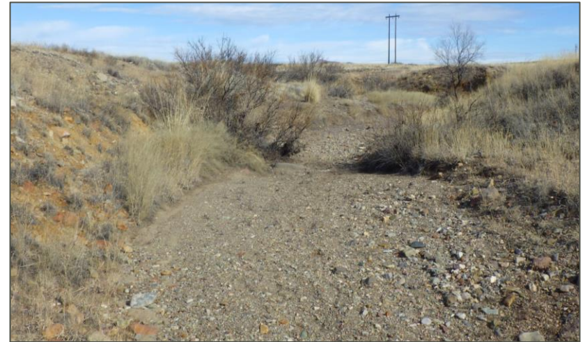
January 2020. General channel conditions. Looking upstream.
