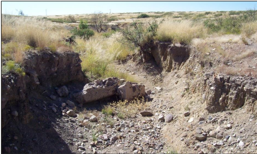
October 2008. West headcut at Edwards Ranch. Looking downstream.
