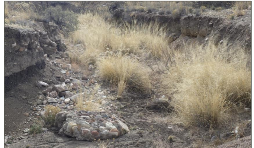
January 2020. West headcut at Edwards Ranch. Looking downstream.
