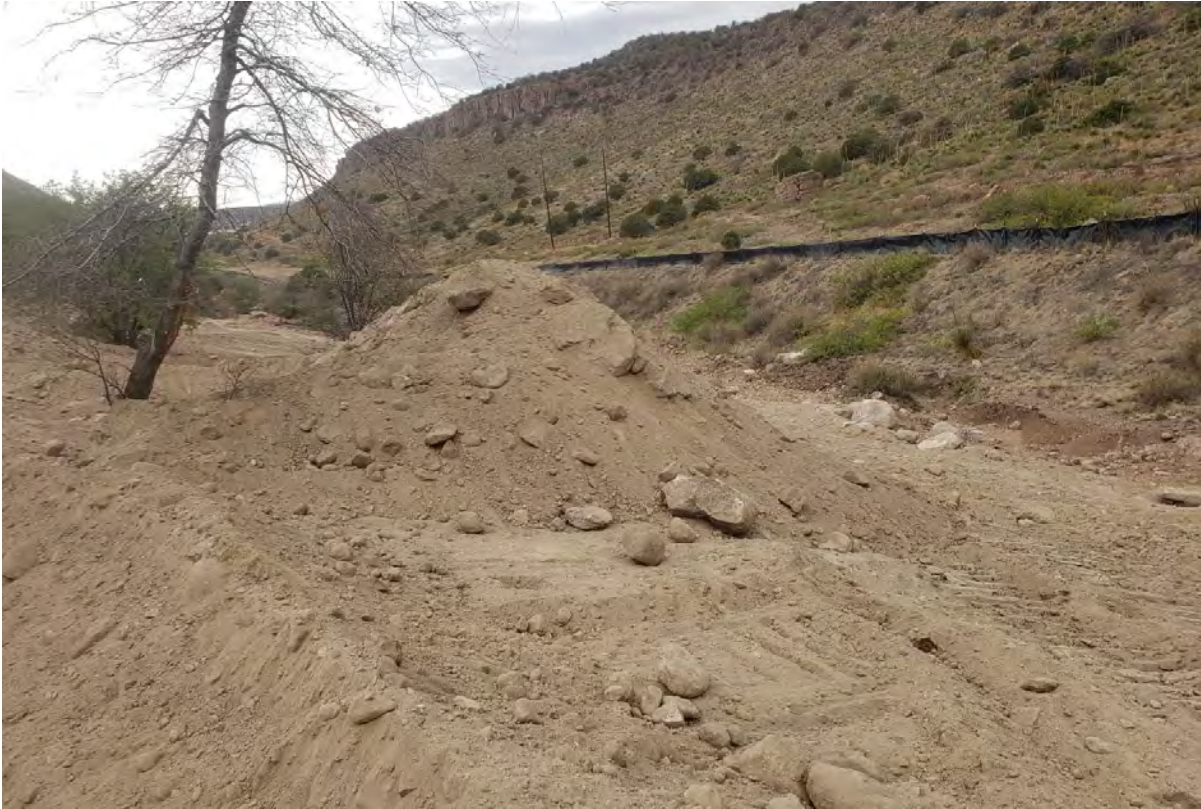
Photo 3: Cover and a mound were placed over Shaft 2.
