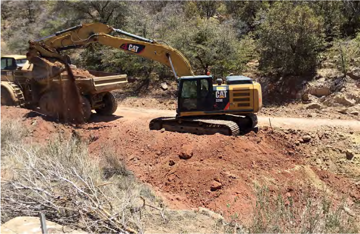
Photo 1: Shared Services removed red material at Shaft 1 along access road.
