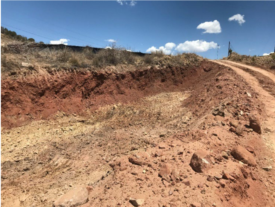
Exhibit 5a – Photograph showing the remaining stockpile left in place under the stockpile and pipeline corridor.
