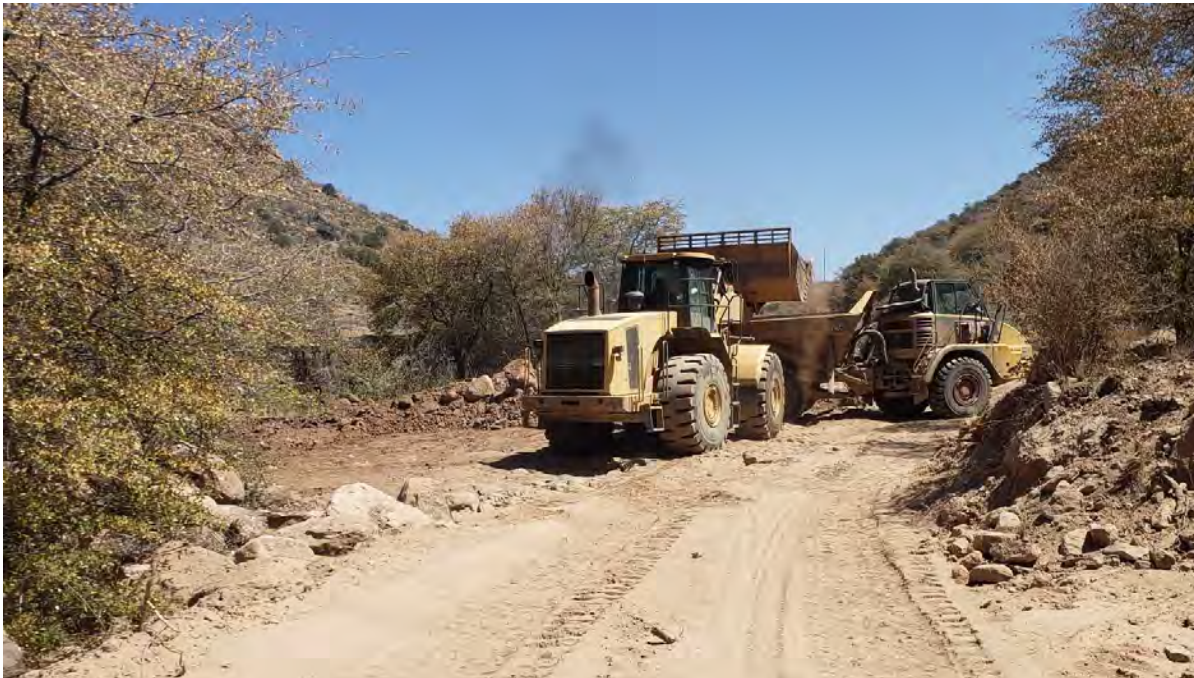
Photo 3: Using loader to remove stockpiles of reddish material across from Shafts 4 & 5.
