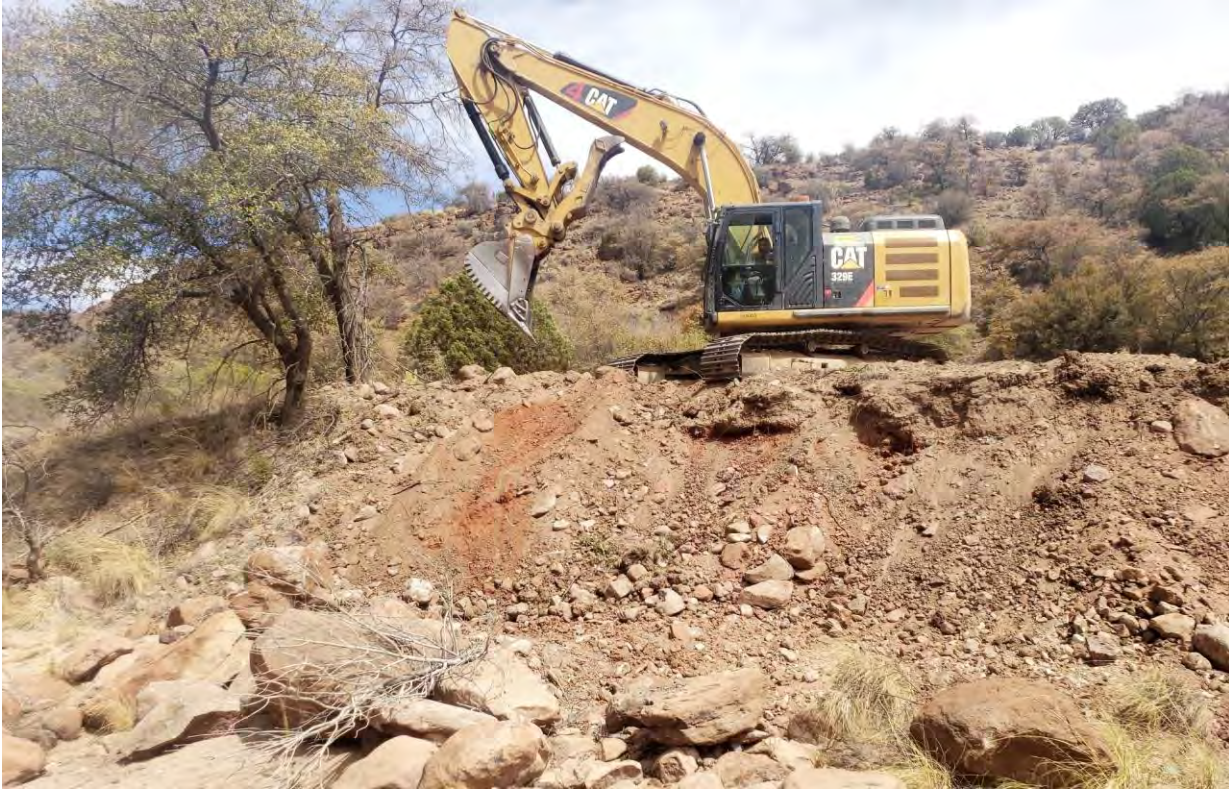
Photo 1: Shared Services removed red material from east bank of creek, adjacent to former mound
