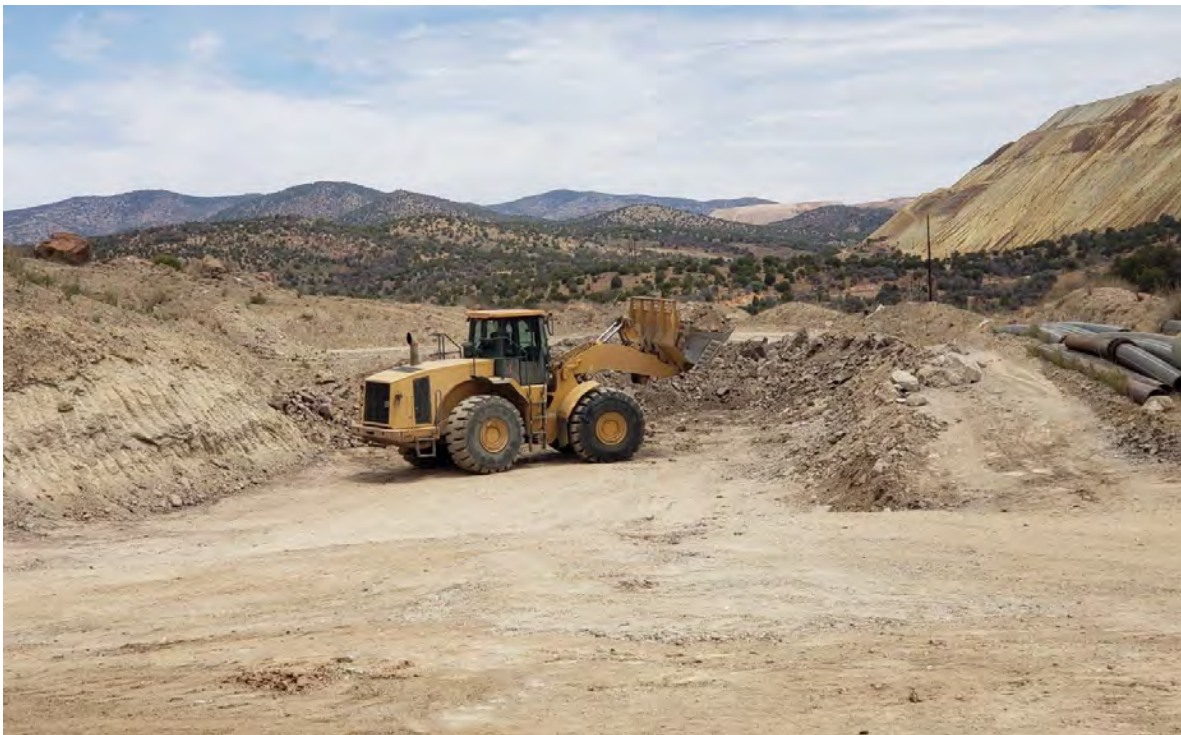
Photo 2: Cover material was loaded from borrow source near former Groundhog Mine.
