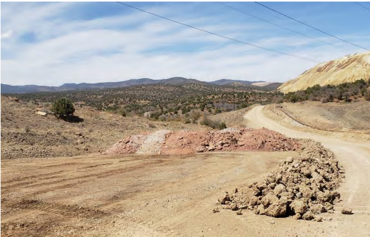
Photo 2: Shared Services built containment berms for a new stockpile and began hauling to it.
