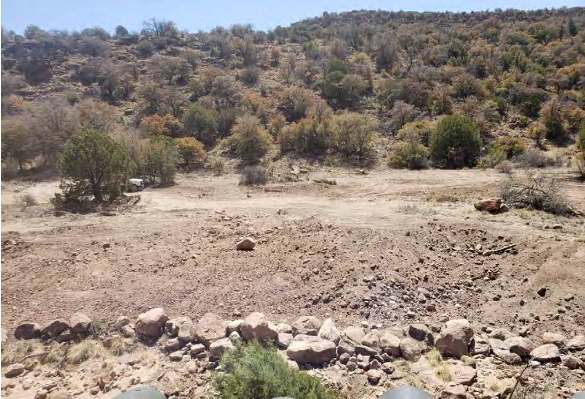
Photo 1: Excavation is complete in large area and creek bank near Shaft 8.
