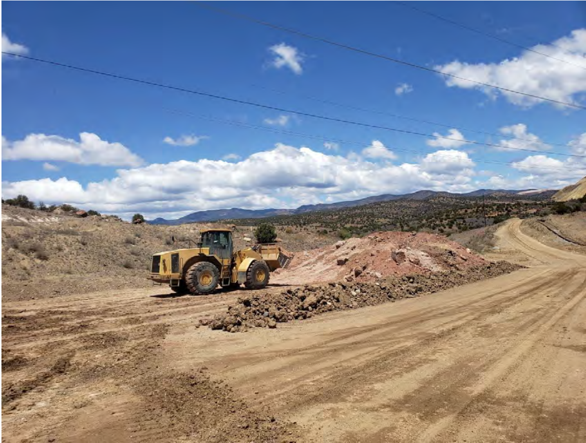
Photo 3: Shared Services consolidated material at new stockpile.
