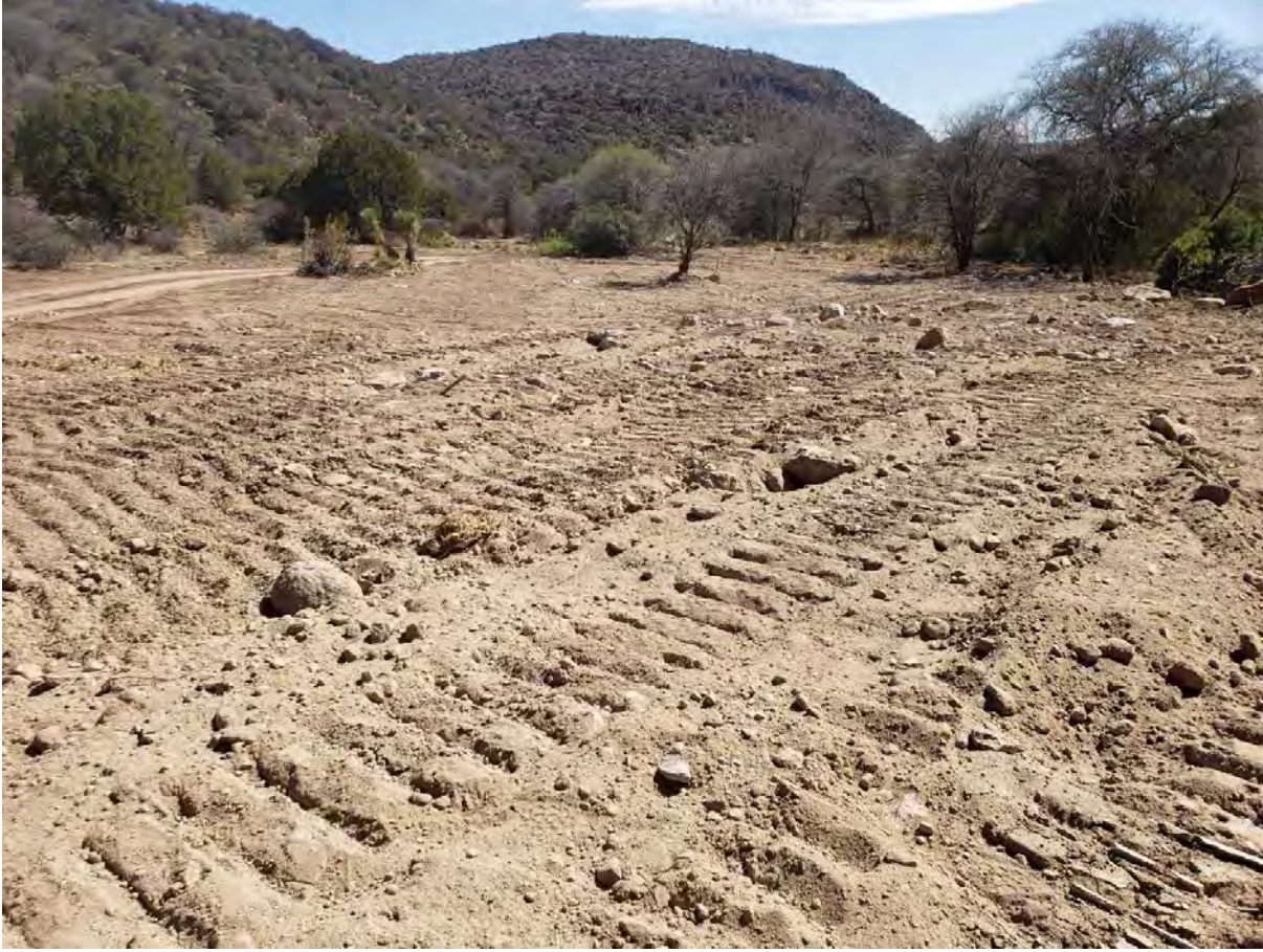
Photo 3: Large areas in the central portion of the site were backfilled and graded.
