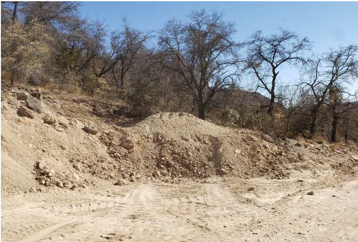
Photo 4: "Ant-hill" mound was placed above former working south of Shaft 2.
