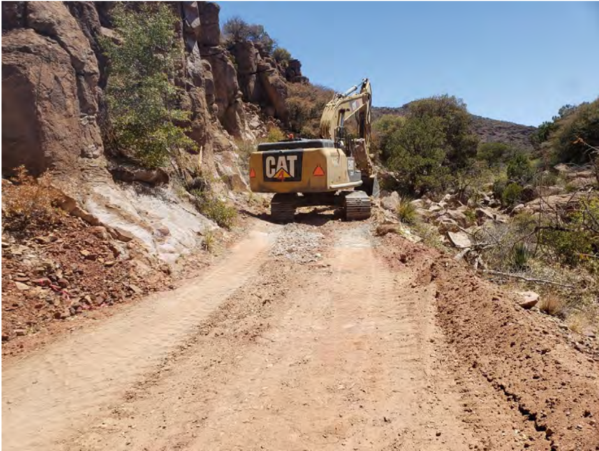
Photo 3: Removal of red, yellow, and gray material comprising road into Lucky Bill Canyon.
