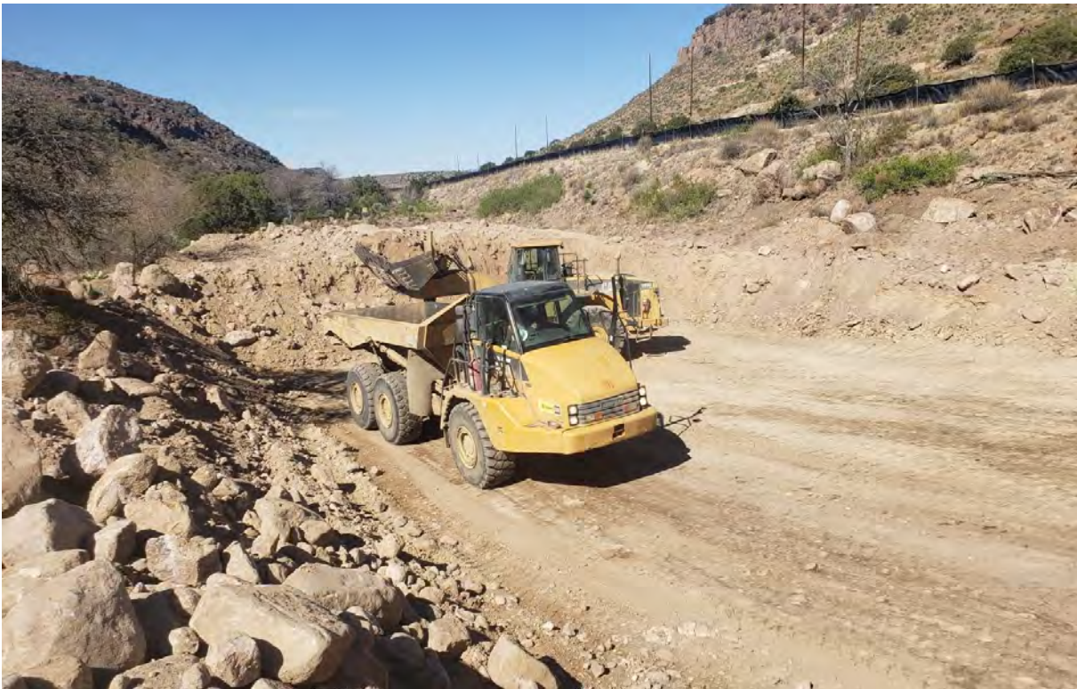
Photo 2: Crew loaded backfill material into haul truck at borrow area.
