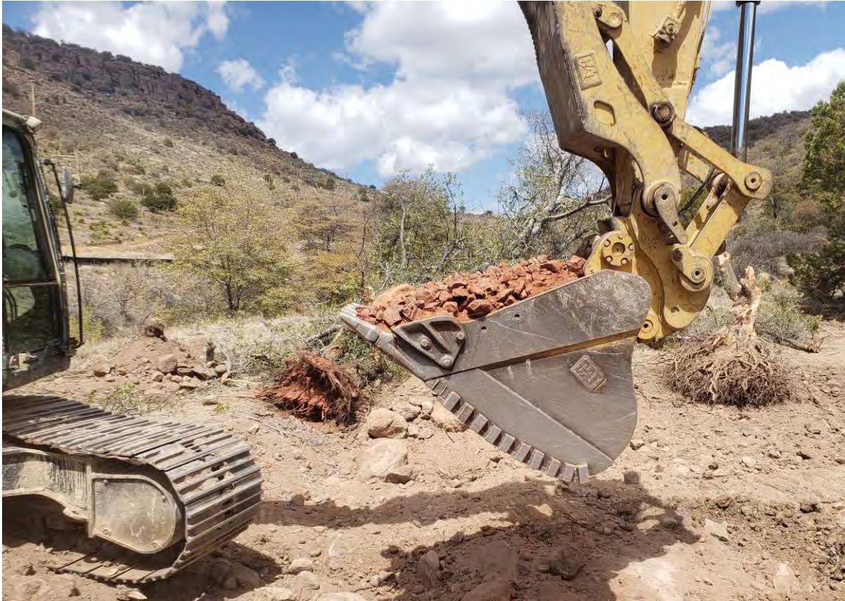
Photo 3: Red material from the creek bank west of Shaft 8 was removed.
