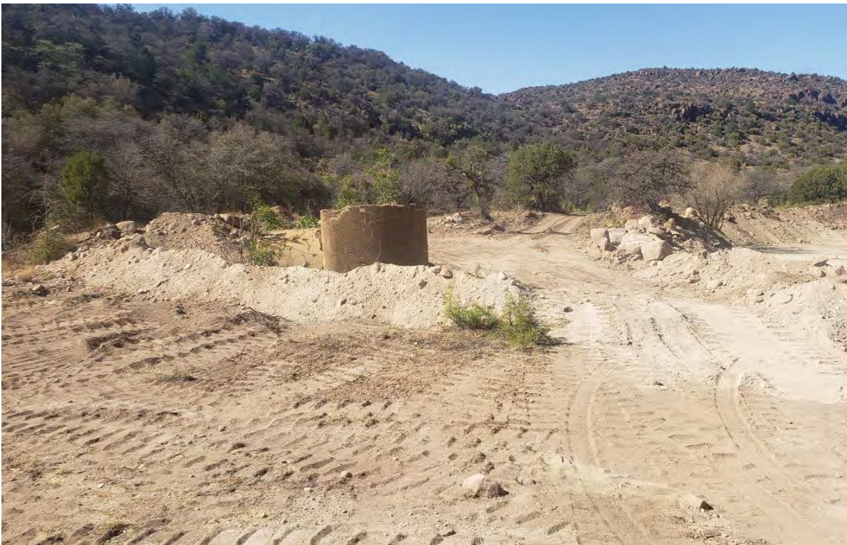
Photo 4: Berms at southern borrow area also prevent stormwater from following access road.
