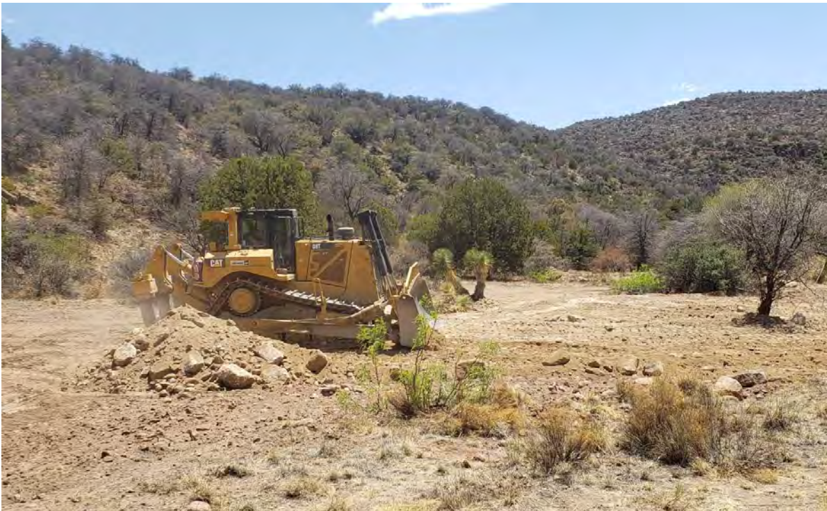
Photo 2: Crew used dozer to grade backfill material into excavated areas.
