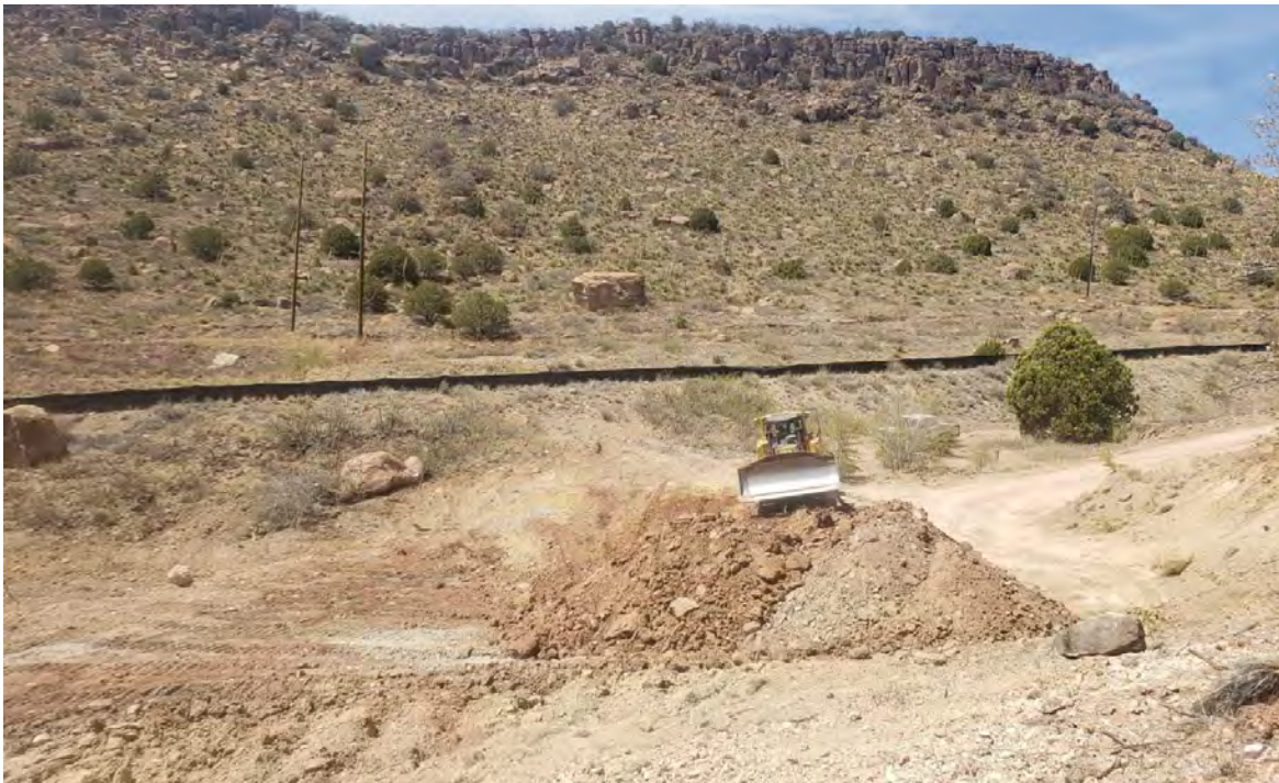
Photo 2: Crew used dozer to push piles of reddish material at removal platform.
