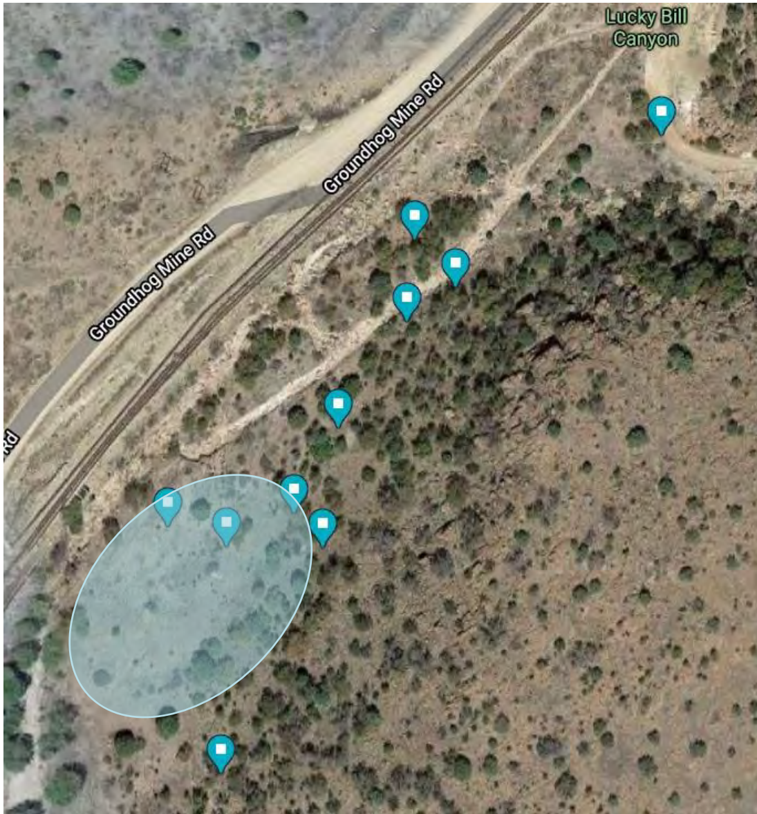
Figure 3: Central Area Backfill Map: Shared Services also started backfill at a large central removal area (blue oval) today.
