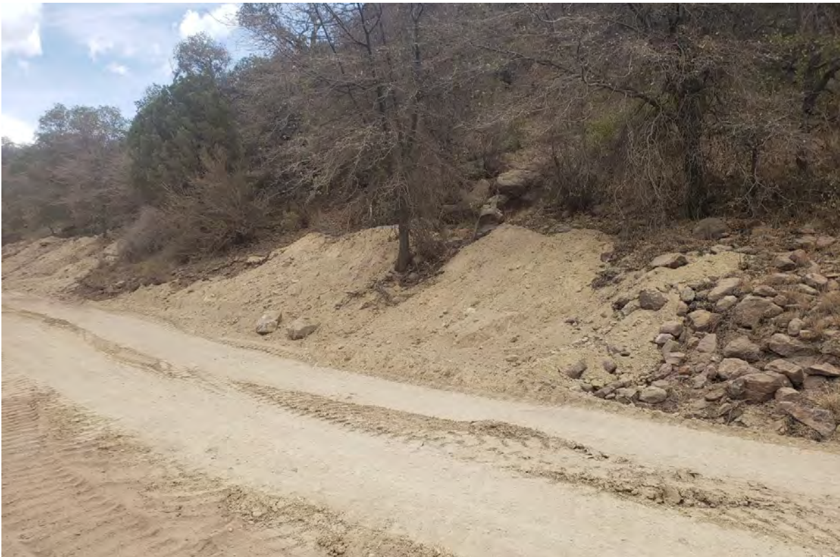
Photo 4: Additional backfill was completed along haul road below Lucky Bill.
