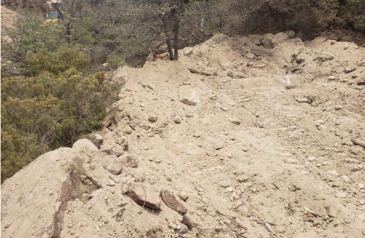
Photo 3: Material was added to reinforce creek bank.
