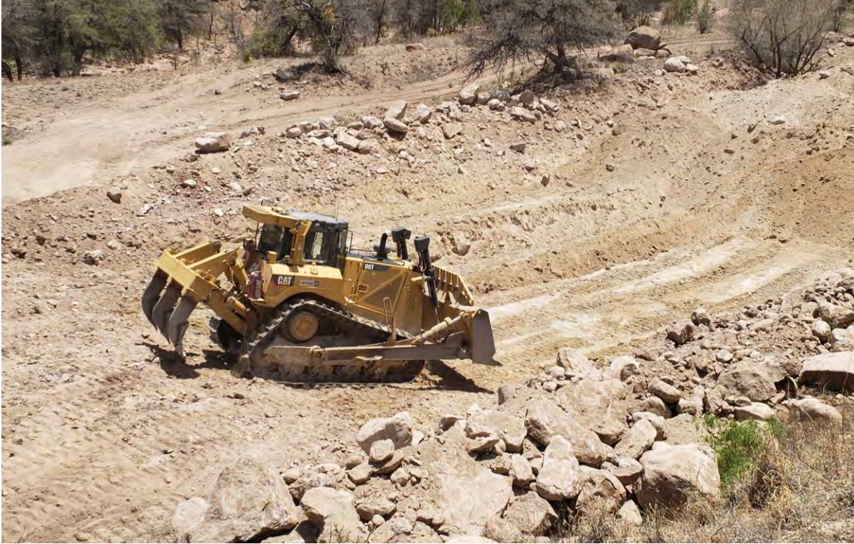
Photo 1: Pete continued dozing and stockpiling cover material at southern borrow area.
