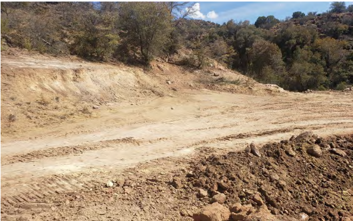
Photo 4: Crew finished excavation of slope leading into Lucky Bill Canyon.
