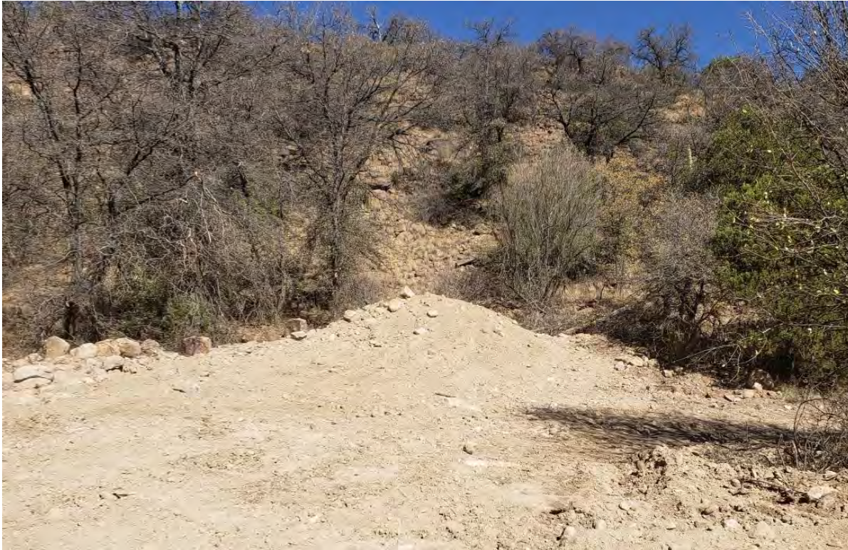
Photo 3: "Ant-hill" mounds were constructed above former workings south of Lucky Bill.
