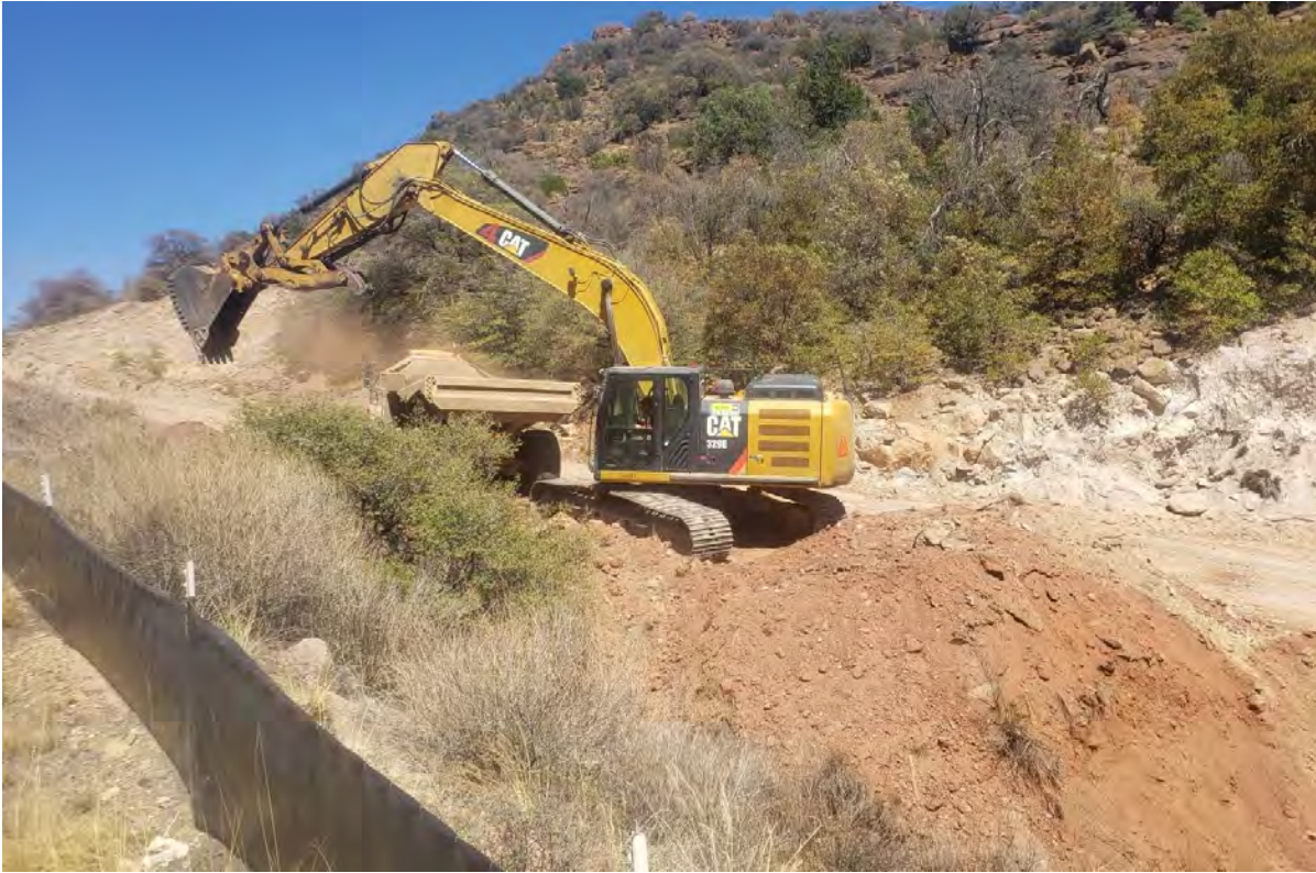
Photo 1: Shared Services removed red material at Shaft 1 along access road.
