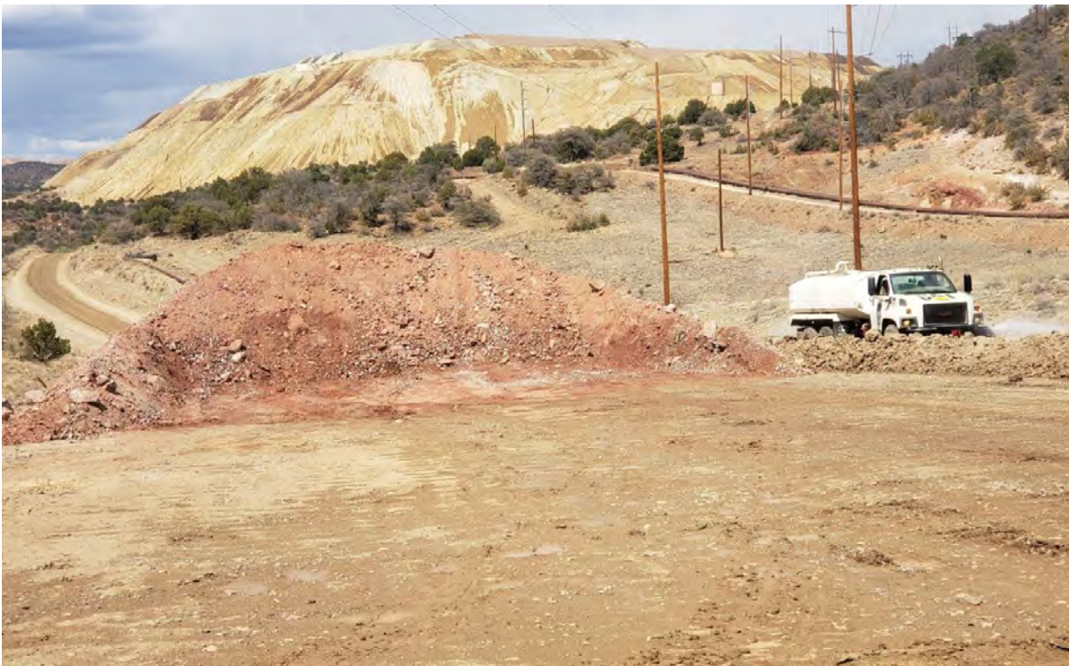
Photo 2: Shared Services used water truck for dust suppression on stockpiles and haul roads.
