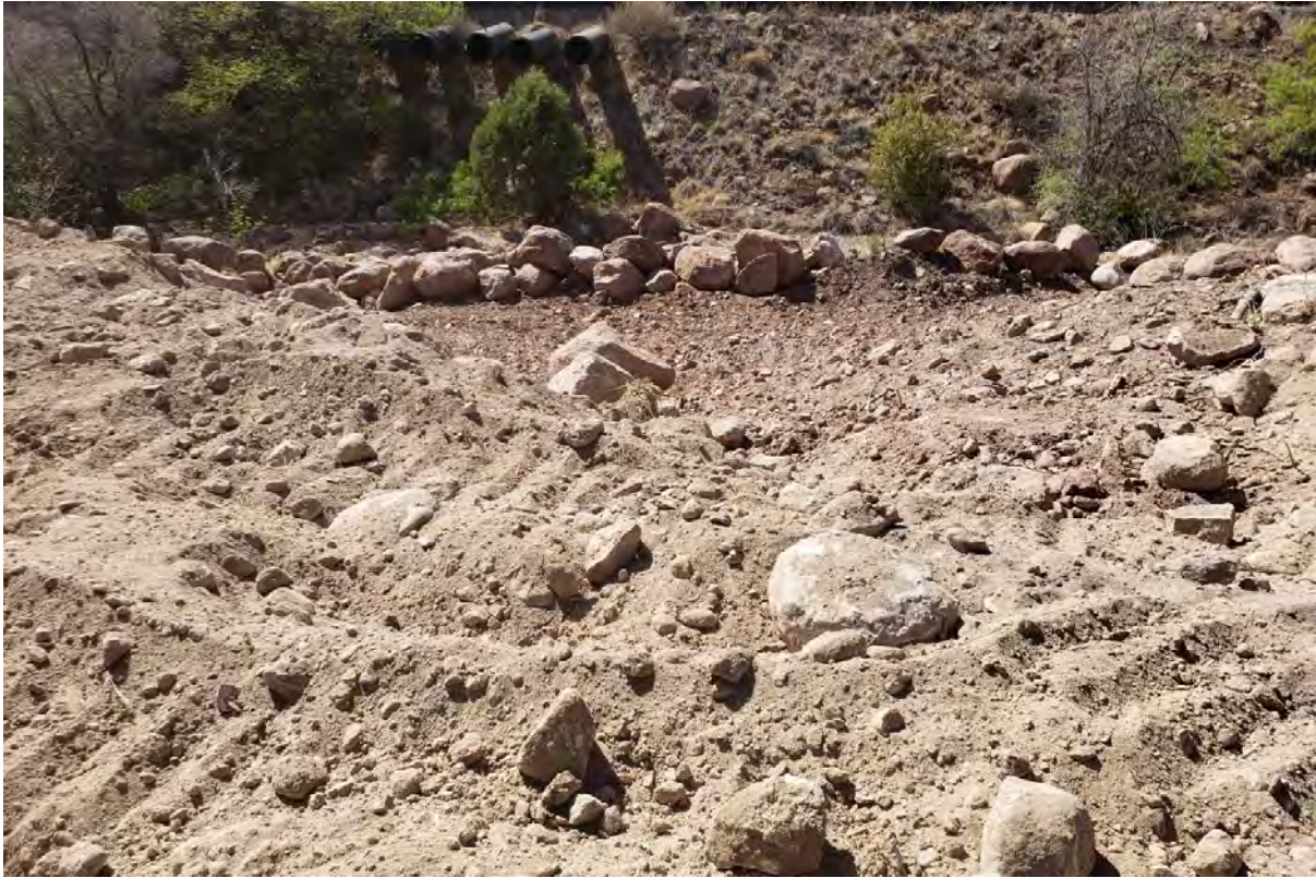
Photo 1: Partially-backfilled areas along creek bank at central portion of jobsite.
