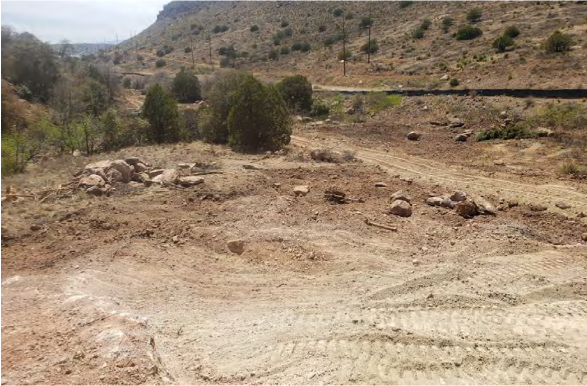
Photo 3: Broad areas SW of Lucky Bill where removal was completed 5/4/21
