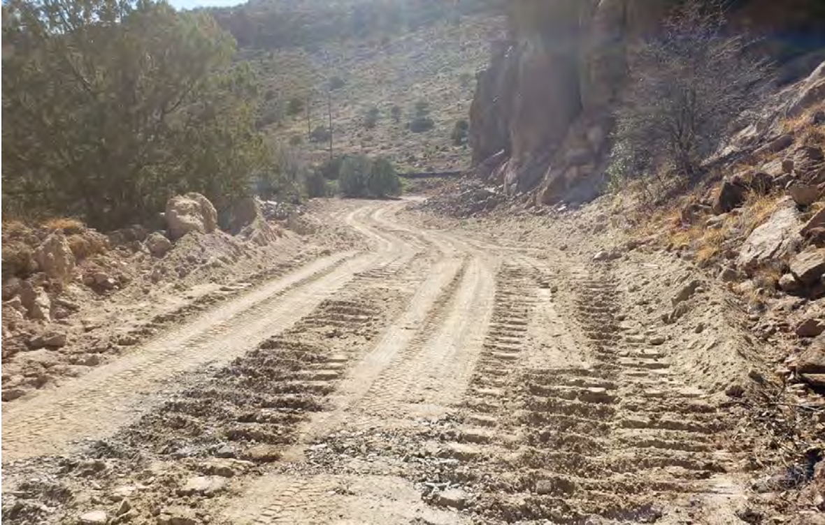
Photo 1: Shared Services nearly finished reconstructing road into/out of Lucky Bill.
