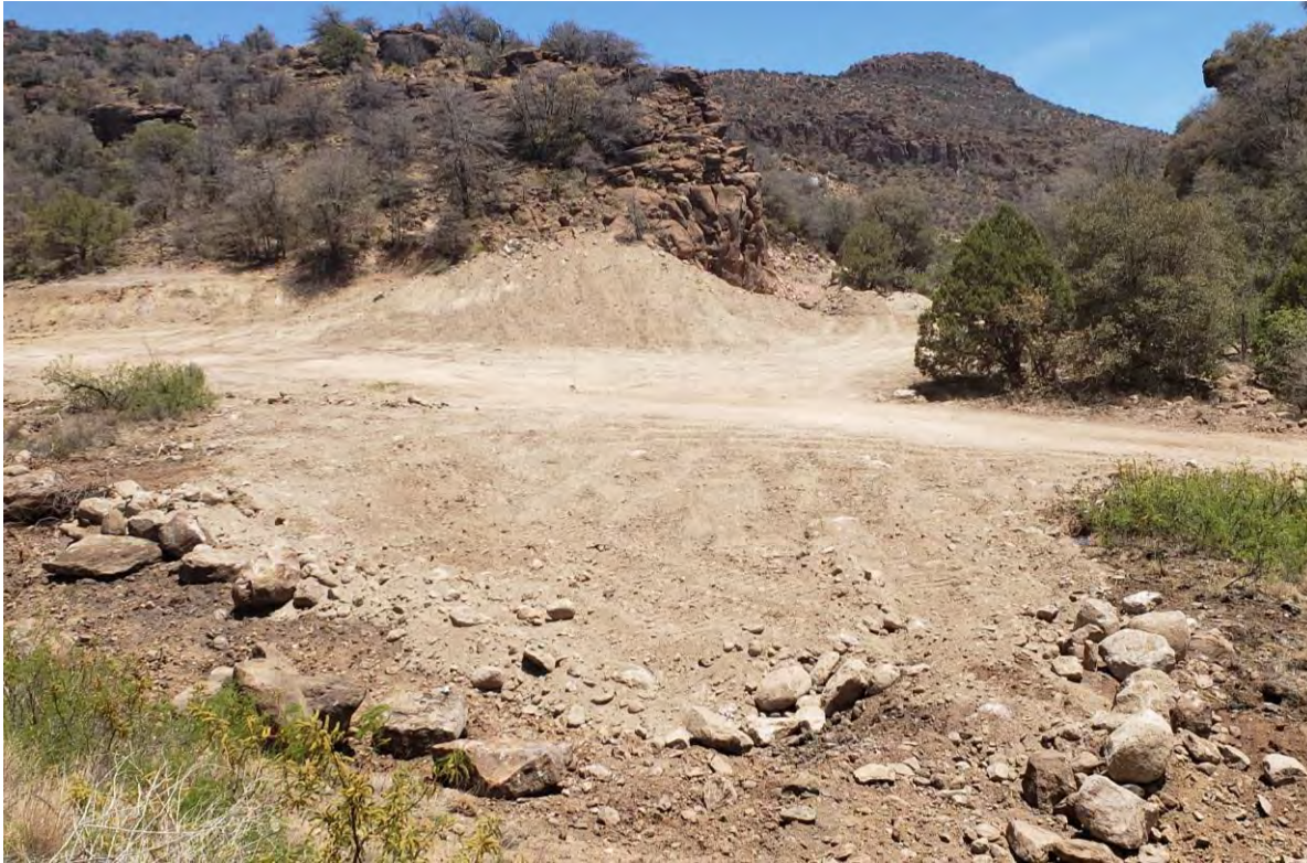
Photo 3: Crew continued backfilling entrance into Lucky Bill Canyon.
