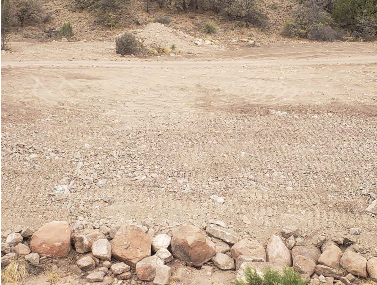
Photo 3: Boulders and rocky cover material armoring creek bank where deep cut was excavated
