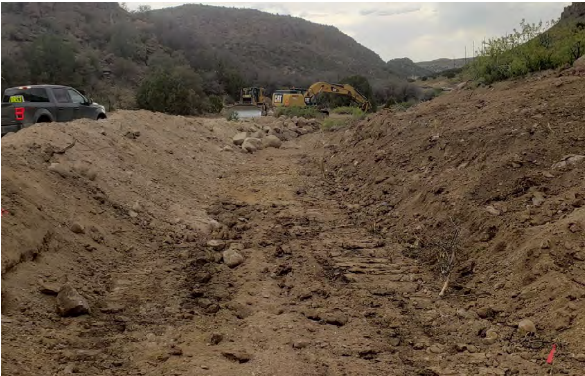
Photo 2: Crew re-cut a channel in the creek bed above Lucky Bill.
