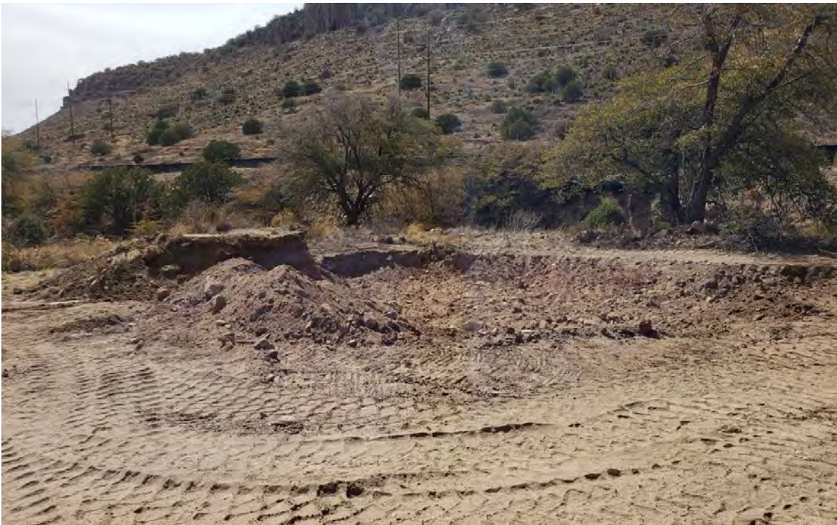
Photo 2: Material beneath a former mound was removed.
