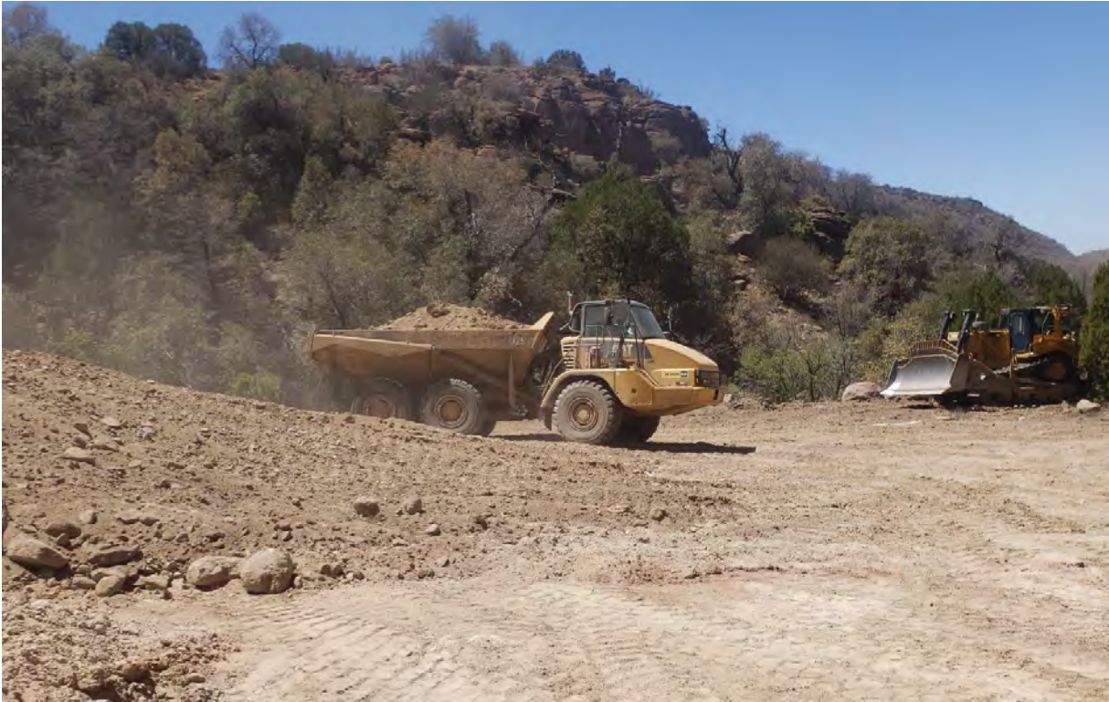
Photo 1: Crew backfilled area and rebuilt road leading into Lucky Bill Canyon.
