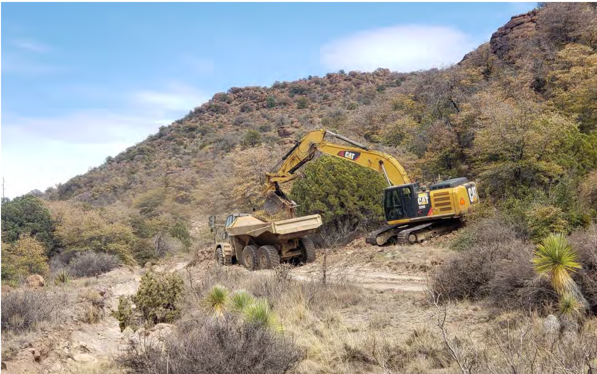
Photo 2: Material from above and around Shaft 6 was removed 4/15/21.
