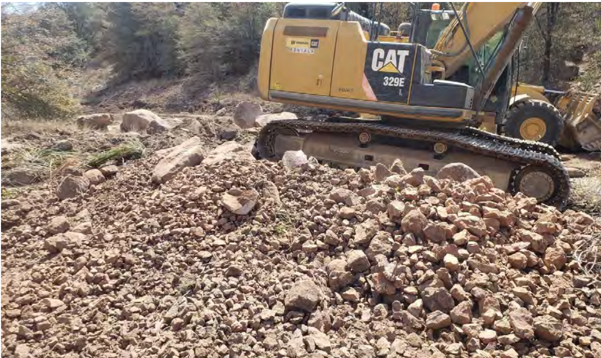
Photo 2: Small stockpiles east of Shafts 4 and 5 were gathered for removal.
