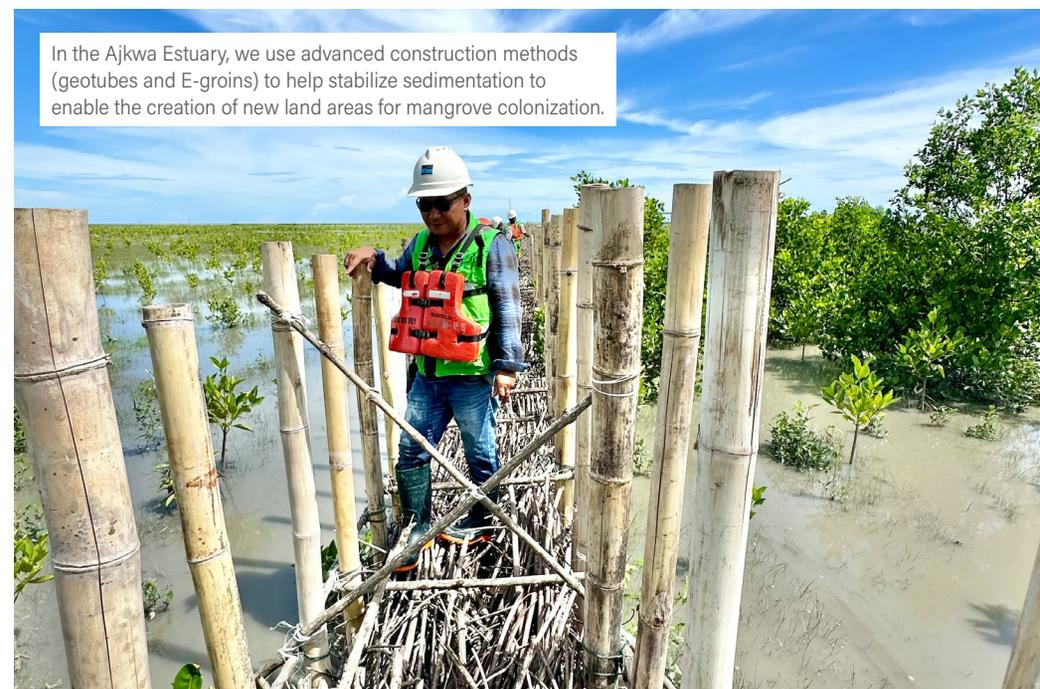
In the Ajkwa Estuary, we use advanced construction methods (geotubes and E-groins) to help stabilize sedimentation to enable the creation of new land areas for mangrove colonization.
